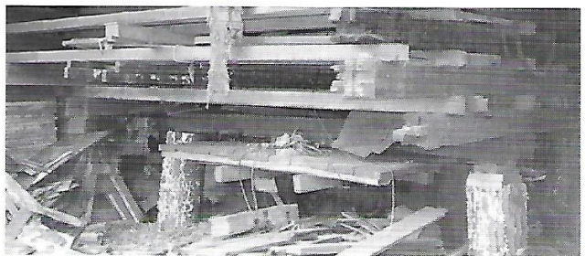
Above: Notice as they jacked the weight off the truck, sections of a log with shims were used to support the building.
